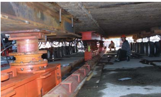
The drydock was mounted on 16 jacks, each with eight wheels, and towed from the barge to Foss Terminal. Ron Becker monitors the towing mechanism.
