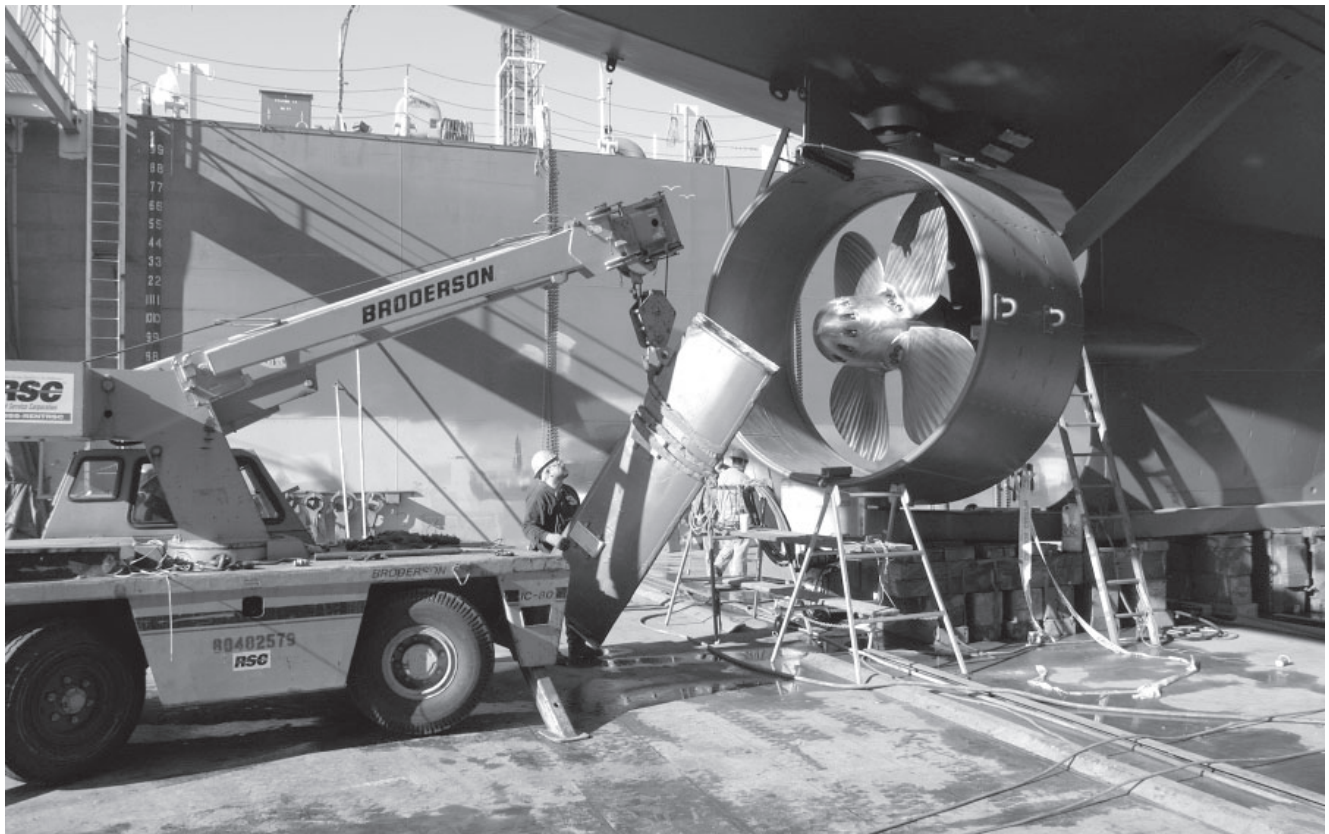
Rigger Assistant Foreman Terry Dawley gets ready to hoist the Wecoma’s “monkey rudder” into position, on mounts attached to the kort nozzle that surrounds the vessel’s controllable-pitch propeller.
