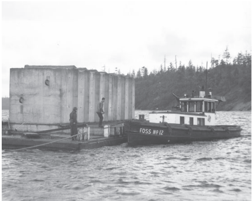
The crew of tug Foss No. 12 prepares to flood the port side of the deck barge to allow the 600-ton cement anchor to slide off into the appointed location in the Tacoma Narrows. (1939)
