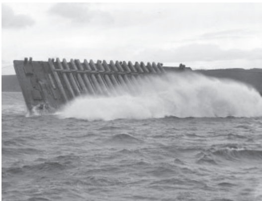
The concrete anchor has just slid off the barge into the Narrows. (1939)
