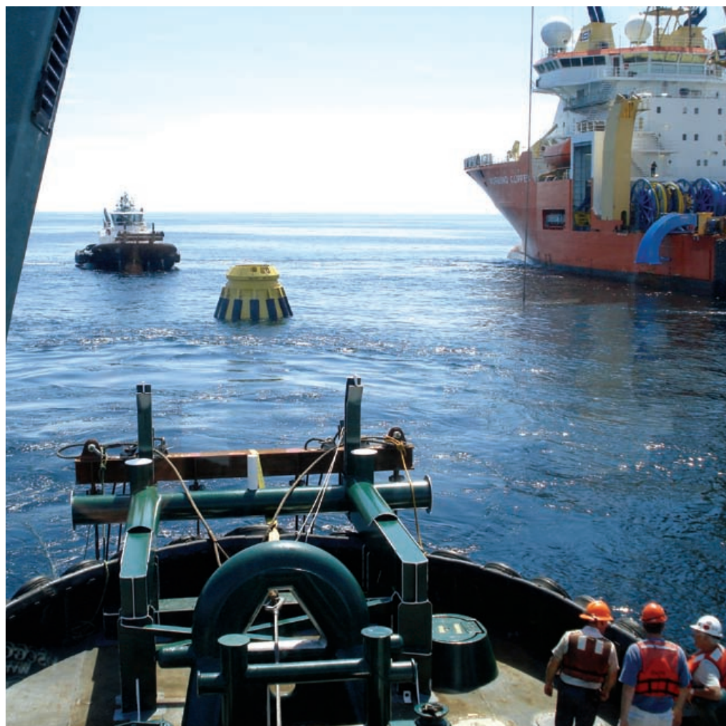
The tractor tugs Orion , in the foreground, and Leo hold mooring wires in place at the LNG terminal site while the wires are attached to anchor chains by a submersible vehicle. Between the two tugs is a 200-ton buoy, which will be submerged, serving as both a mooring for ships and a conduit for their cargo.
