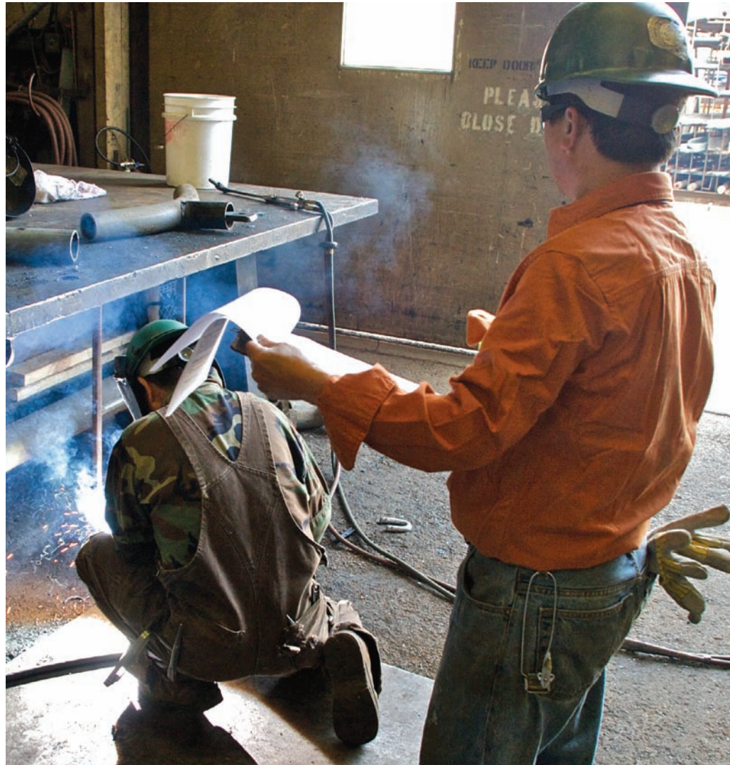
Welder Meang Kang works on a piece of pipe as Linh Tran observes in the steel shop at the Seattle Shipyard.
