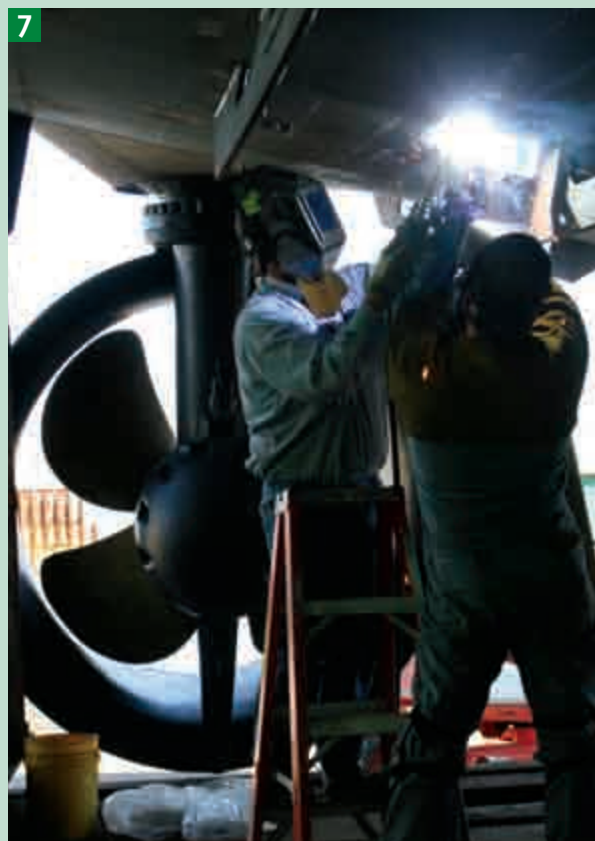
7 Welders work on the tug's bottom, with a newly installed Z drive in the background.
