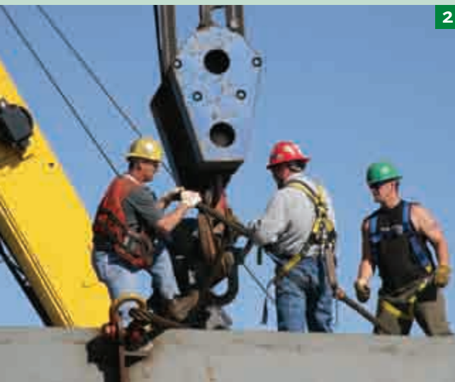
2 Rainier workers adjust the rigging on the stern section before it is lifted for its short upriver voyage.
