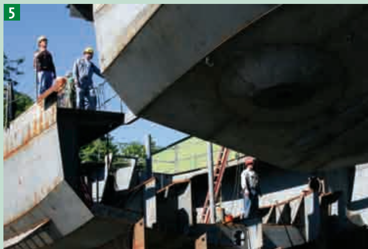
5 Workers guide the stern for the last few feet, soon to find out that it fit perfectly with its partners.
