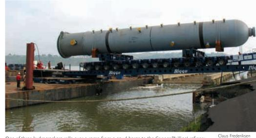
One of three hydrocrackers rolls over a ramp from a spud barge to the ConocoPhillips' refinery.
