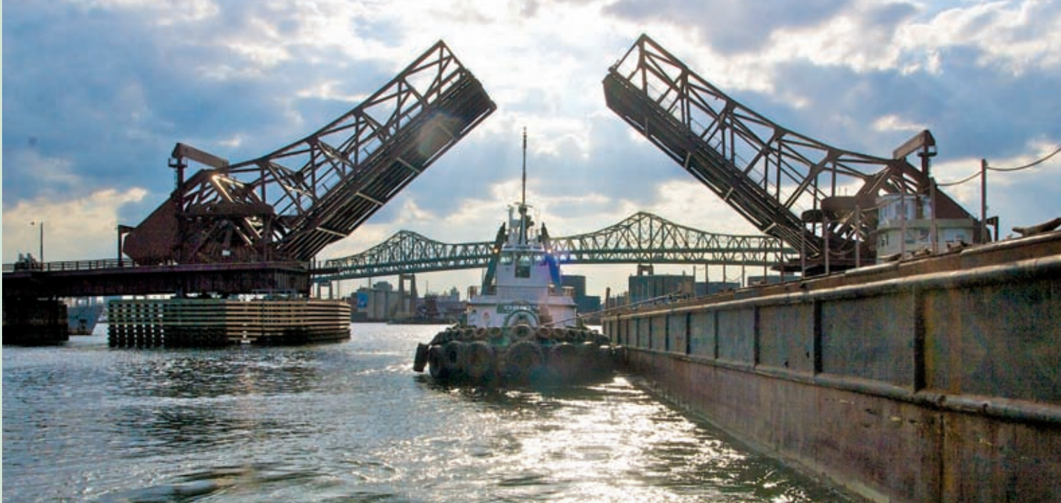
With the Orion in the lead, the barge Chem Caribe heads for the narrow opening of the Andrew McArdle Bridge at the opening of the Chelsea River.
