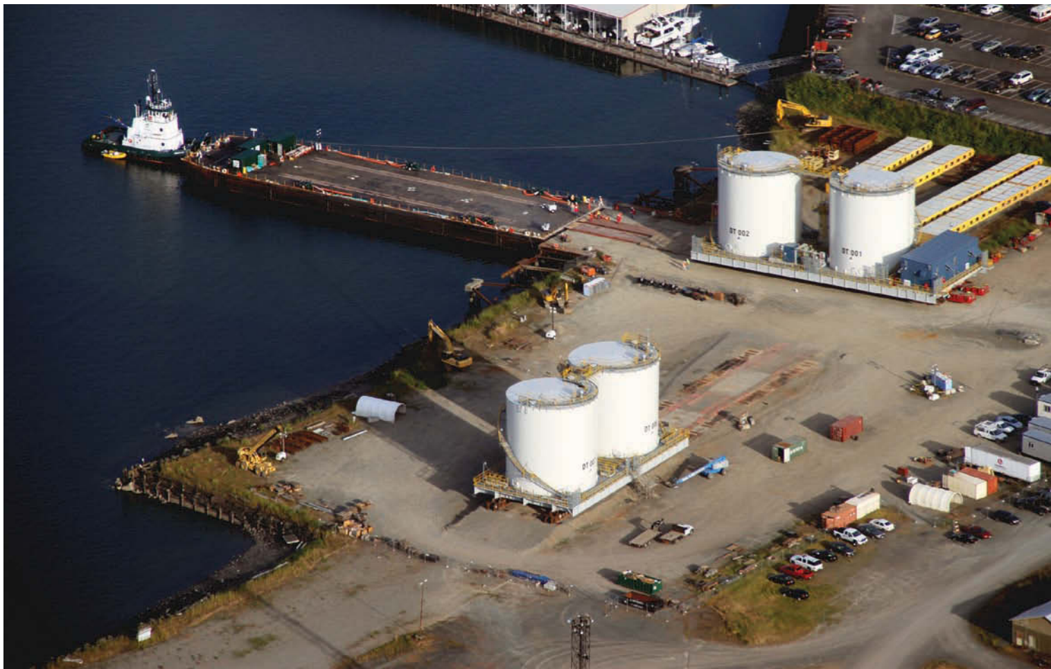
The first two of four large oil tank modules were ready to be loaded onto a barge in Anacortes, Wash.
