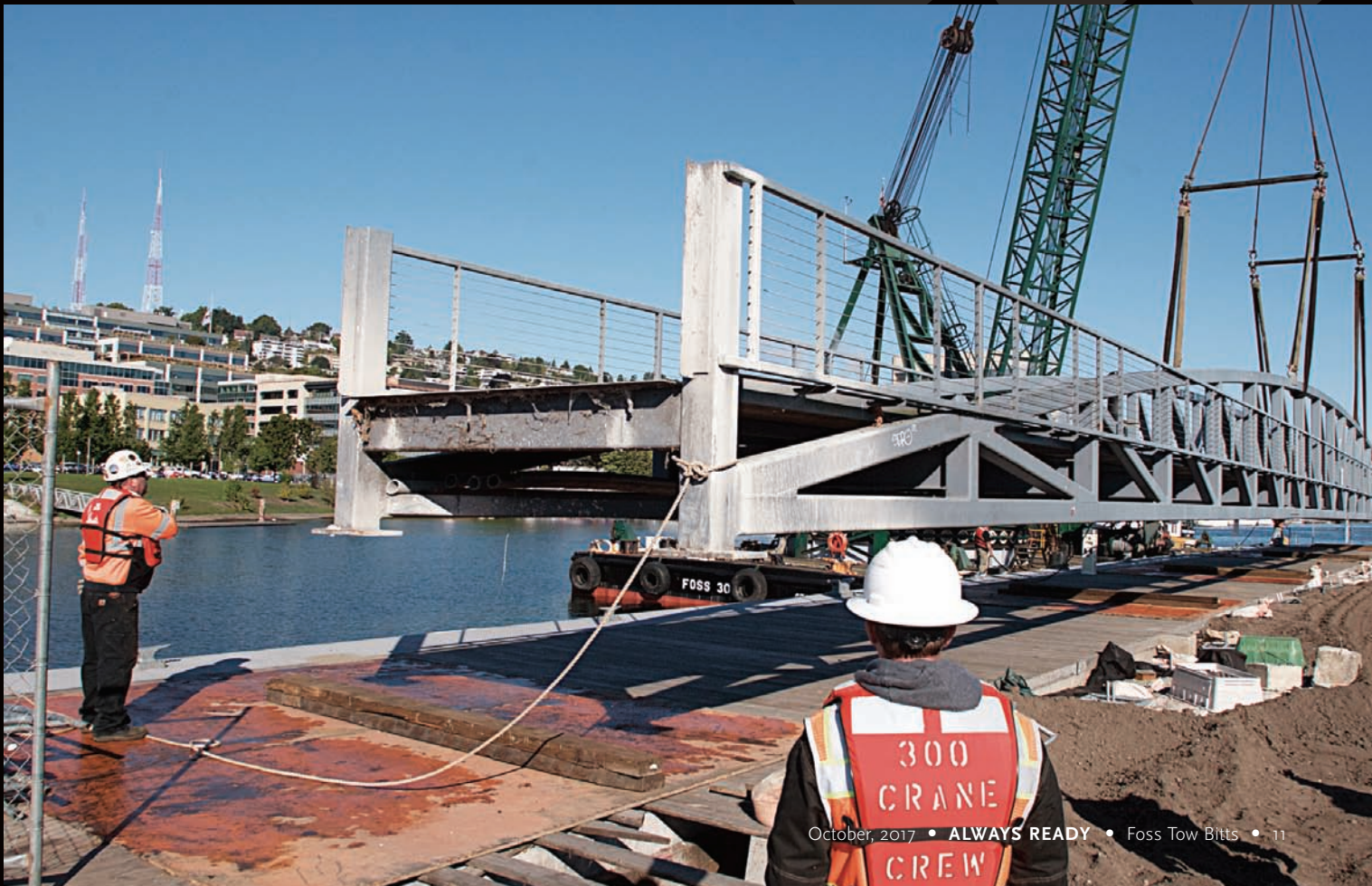
5. Below: The floating crane sets the bridge down on the pier. John Tarabochia, left, supervised the job for Foss.
