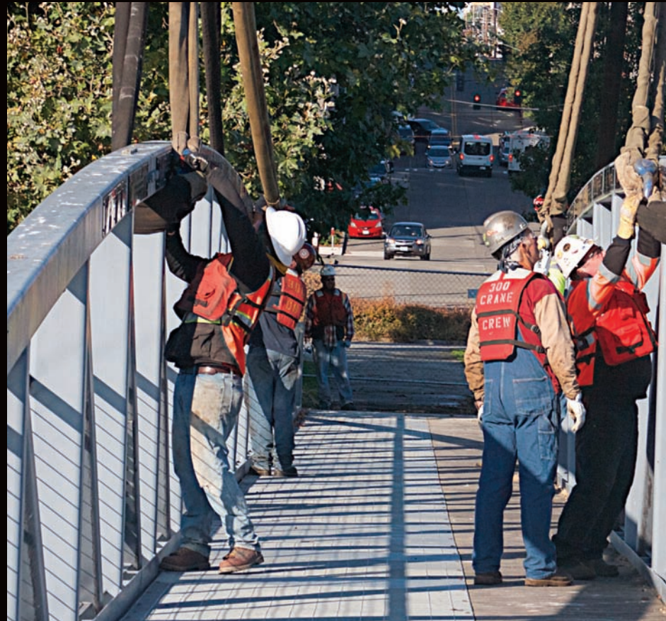
3. Below: Hard-hatted workers rig the Lake Union Park Bridge for the lift.
