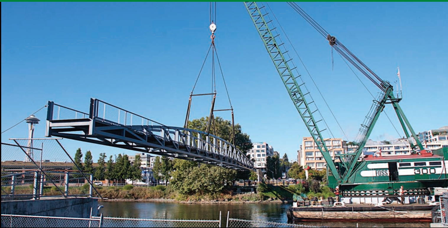
4. Above: The bridge rises over the lake as the Foss 300 lifts it from its abutments. Note the Space Needle in the left background.
