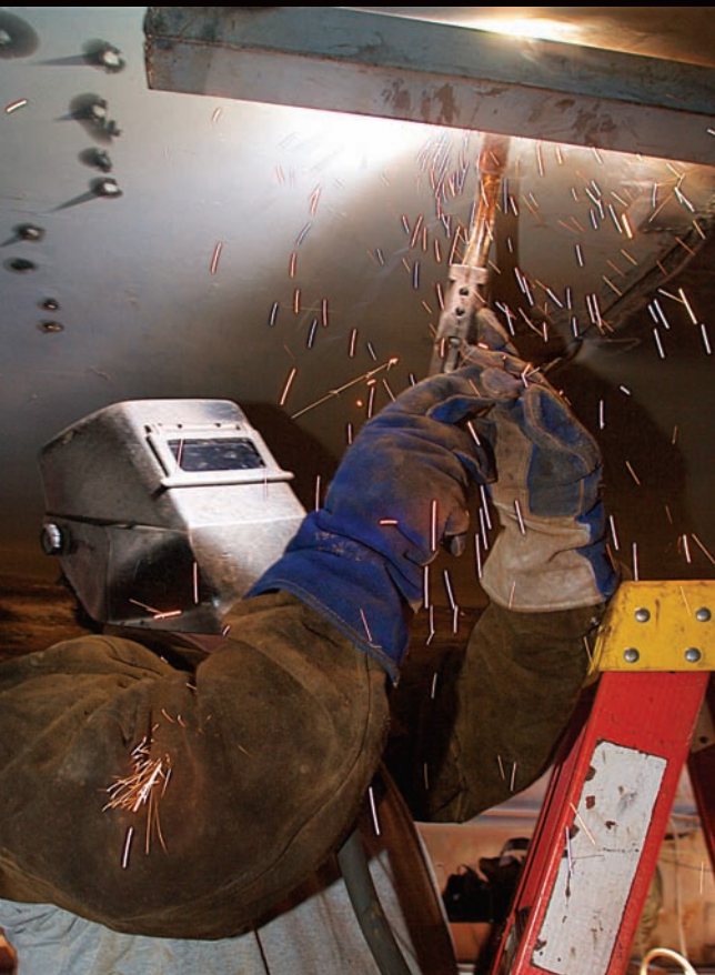
2. Below: Welder Nery Barrientos works on the hull of the historic barge crane.
