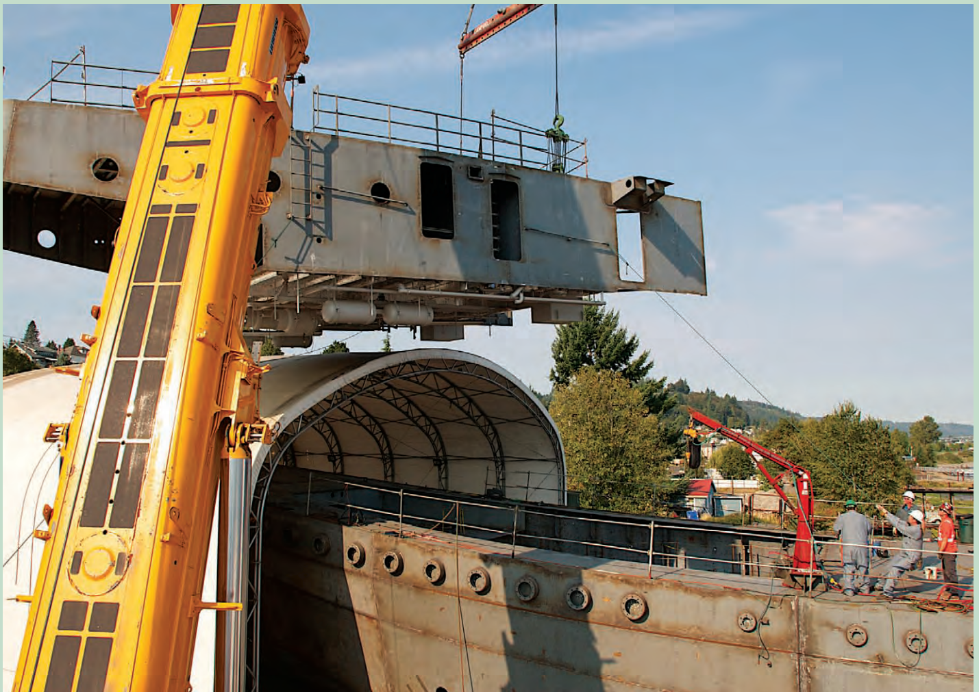
DENISE HAS A HOUSE The lower portion of the house, at 85,000 pounds, was lifted aboard the Arctic-class tug Denise Foss in early September at Foss Rainier Shipyard in Oregon. The tug is the second of three ocean tugs being built at the yard. More photos appear on page 17.
