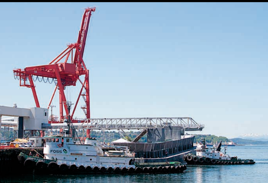
▲ 1. The Sidney Foss , foreground, and the Pacific Knight stand by at Seattle's Pier 46 as an overhead conveyor system loads the tunnel spoils onto a barge for transport to Mats Mats Bay.
