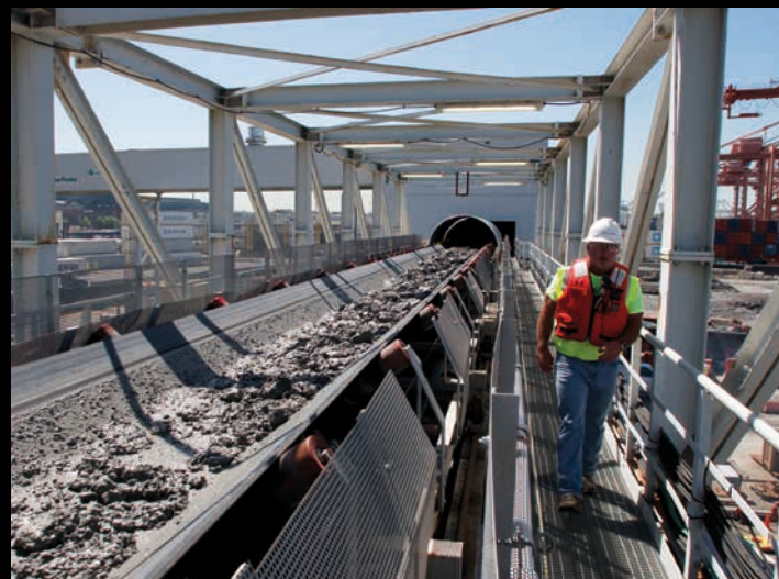
▲ 2. Thomas Nixon is overseeing the barge loading operation. The conveyor system, at left, carries the muck from tunneling machine Bertha to the barge.
