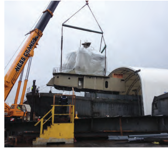
The house was mounted on Feb. 10 on a fireboat under construction at Foss Shipyard in Seattle for the Port of Long Beach. The boat is scheduled to be completed in June.
